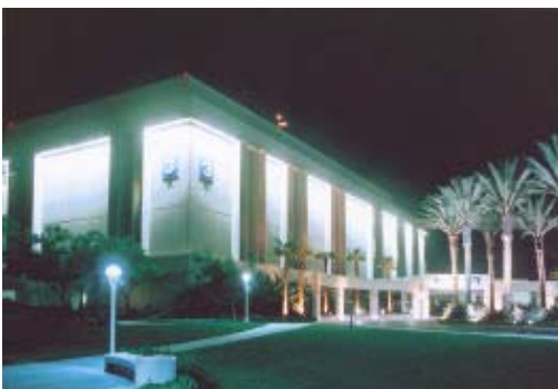
Figure 7.6 - Architecturally integrated lighting can illuminate façade and provide area lighting for building
