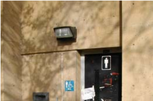
Figure 2.1 – Wall pack with prismatic refractor – visible lamp partially blinds pedestrians.
