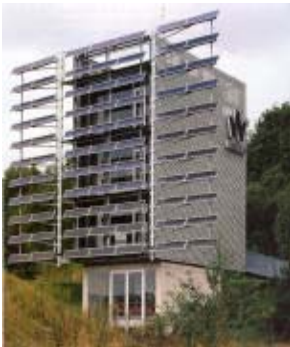
Figure 13.4 – Solar panels can serve double purpose as sun screens for building interiors.
