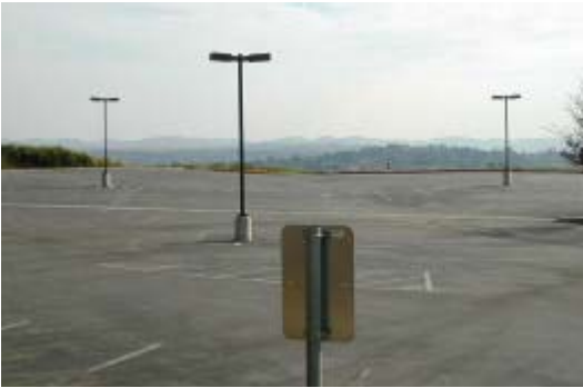
Figure 1.2 – Child Development parking – Low, sparse fixtures inadequate for area of parking lot.
