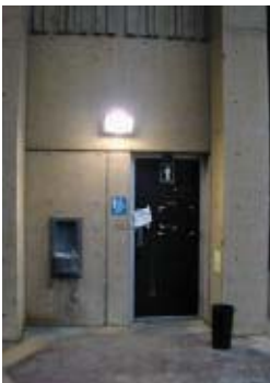
Figure 7.2 – Highly visible glary fixtures are not recommended because they actually reduce visibility.
