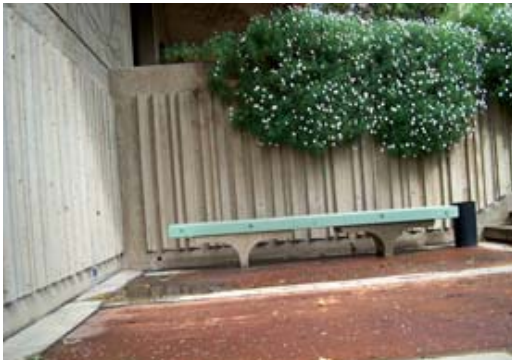
Figure 6.2: Backless concrete bench with painted wood seat located at stair landing. Bench is similar to PAC Plaza benches.
