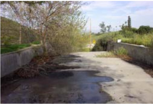
Figure 5 – Retention basin spillway looking westerly downstream to Sand Canyon Road.
