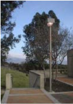
Figure 5.1 – Where pole lights are located at tops of stairs, they can be sources of glare for those ascending.
