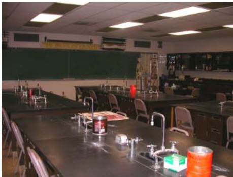
Lab 225 - Non-compliant seating and fixtures; low light levels.
