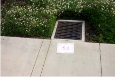
Figure 1 - Typical site catch basin that collects surface drainage.
