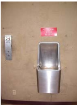
Inaccessible drinking fountain
