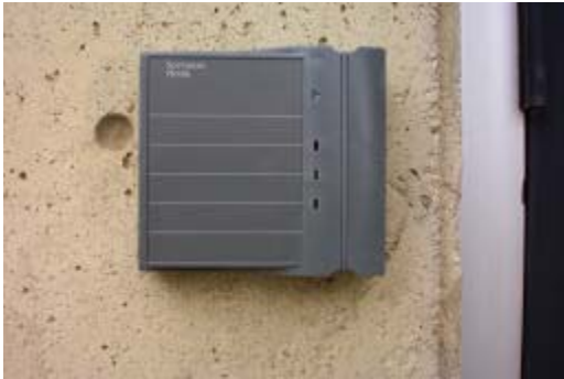
Figure 1 – Proximity Card Reader, (wireless), without keypad. Only addressed with a radio frequency interface card.
