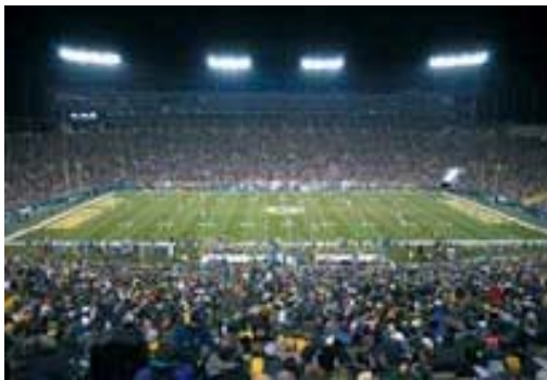
Figure 11.2 – Sports lighting fixtures can be arrayed on poles on both sides of the field to provide even illumination.
