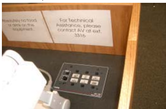
Figure 2 – Push button AV control panel at instructor station allows for equipment selection and volume control.
