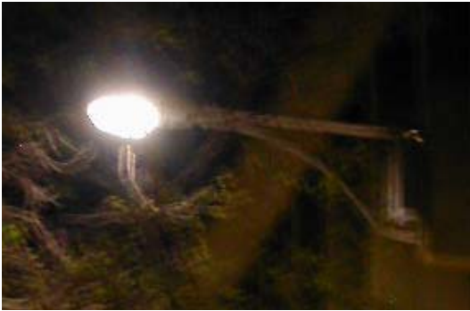
Figure 9.2 – Fixtures cannot store enough energy to last entire night during the winter.
