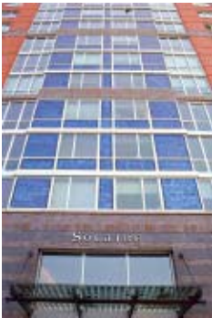
Figure 13.3 – Solar panels can be integrated into building facades, hidden in plain view.
