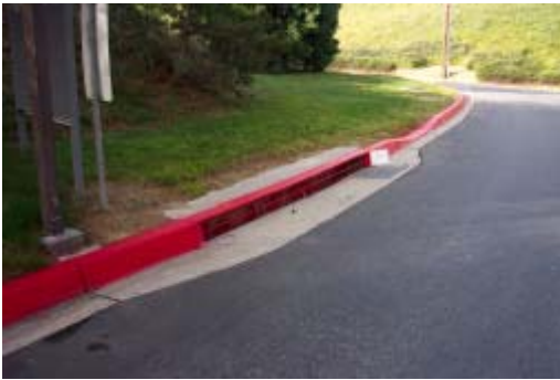
Figure 2 - Typical curb inlet located along Campus Drive.
