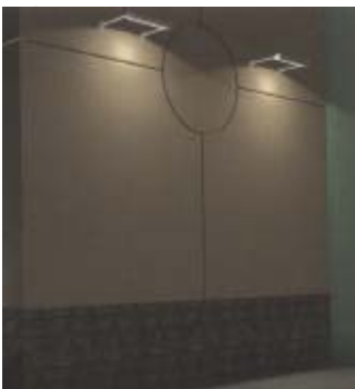
Figure 7.7 - Fluorescent billboard type fixtures can illuminate architecture as well as provide area lighting near
