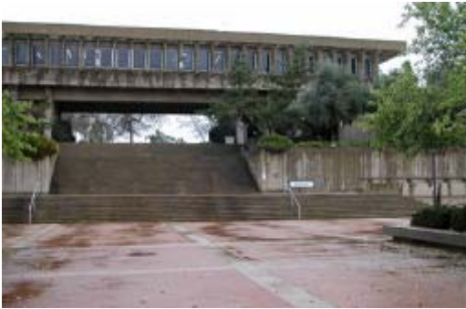
Figure 1 – View of Laboratory/Administration building.
