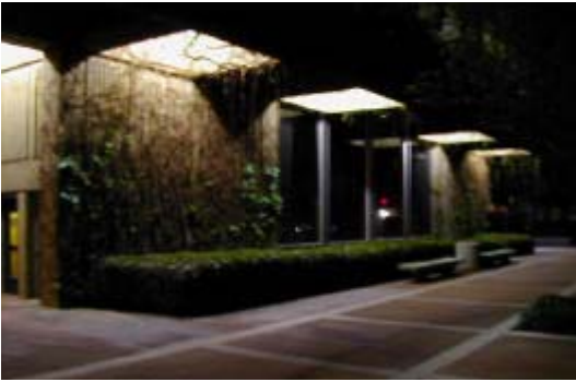
Figure 4.2 – Building integrated lighting serves to illuminate building as backdrop + surrounding.
