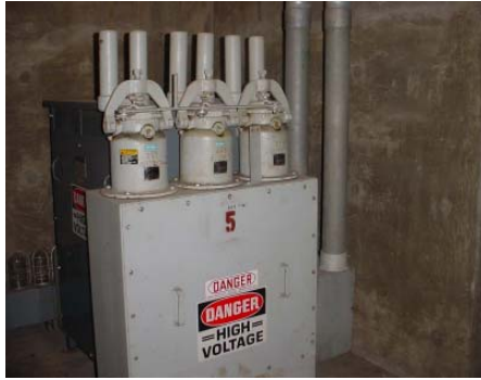
Figure 1 – Oil-filled fuse cut-outs for T-5
