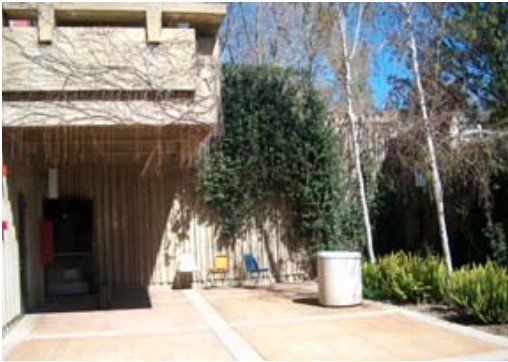
Figure 5.6 View of Foyer space at a SSA classroom entry.
