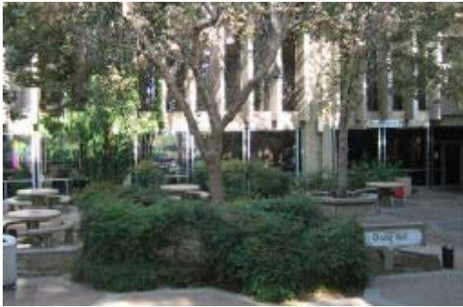
Figure 1 – View of Student Center/Cafeteria building.
