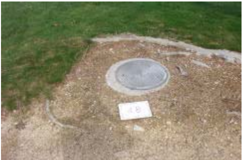
Figure 9 – Typical sanitary sewer manhole located in landscape area.
