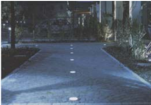
Figure 2.7 – In-grade paver lights help define pedestrian path of travel.
