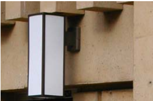
Figure 3.3 – New wall sconces – These use fluorescent, for moderate to good color rendering.
