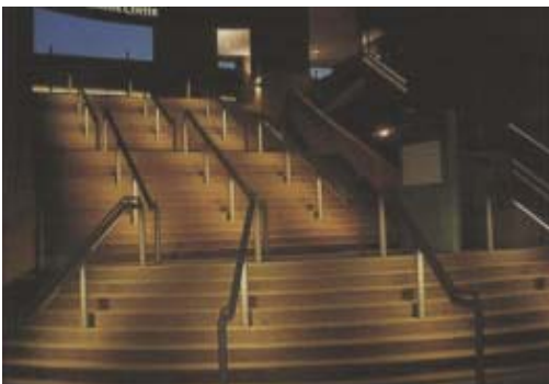
Figure 5.7 – Handrail integrated lighting can provide high levels of glare-free illumination.
