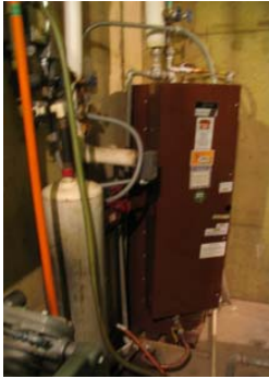
Electric water heater
