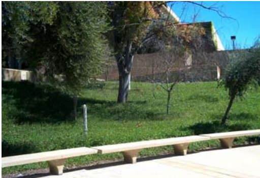
Figure 6.1: Backless concrete benches line the perimeter of the Performing Arts Center Plaza.
