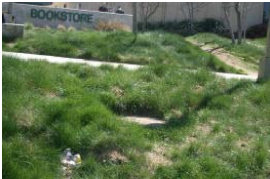
Figure 2 – Manhole location at bookstore is the southern end of campus communications infrastructure spine.
