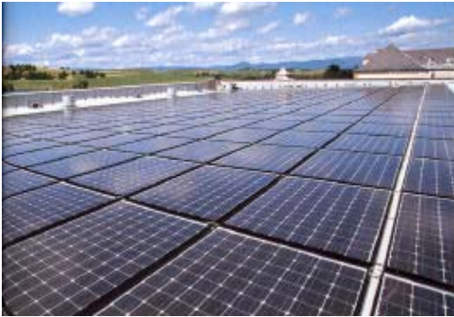
Figure 13.1 – Solar panels can be concealed atop roof tops and aimed for optimal energy collection.
