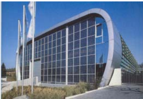
Figure 13.2 – Solar panels can be integrated into building facades, hidden in plain view.
