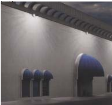
Figure 7.8 - Metal halide cut-off fixtures can illuminate architecture as well as provide area lighting near buildings.
