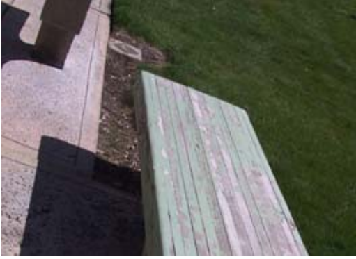
Figure 6.4: Paint and wood wear on many of the existing benches.
