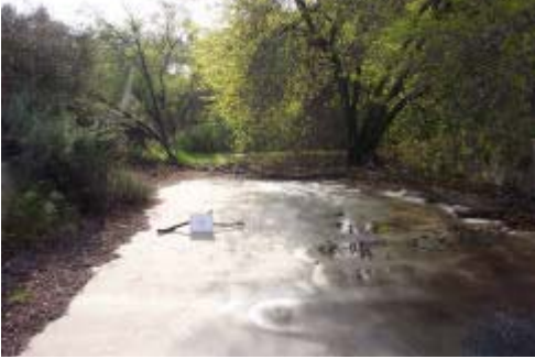
Figure 4 – Retention basin spillway looking easterly into the basin.
