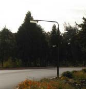
Figure 1.1 – Street lighting - restricted height and wide spacing lead to uneven lighting.
