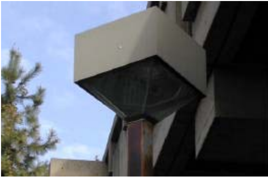
Figure 2.2 – Post top at top of stairs – Pedestrians see into fixture when ascending stairway.
