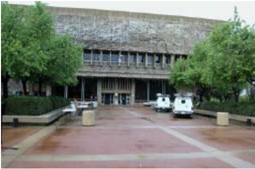
Figure 1 – View of Library building.
