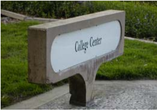
Figure 10.1 – Existing building signage is internally illuminated, although unevenly.
