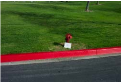
Figure 14 – Fire department connection for the fire sprinkler system for the gymnasium.
